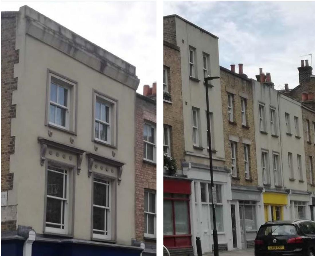
Staining is highly visible on rendered facades due to the pale paint finish.
